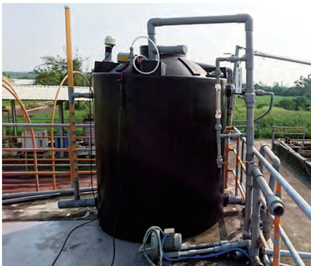
▲簡易之深槽曝氣水洗槽
