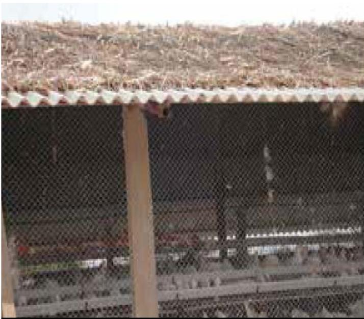
*Figure 8. Use of thatching material (paddy straw, corn stalks, sugarcane tops) to reduce solar heating*
